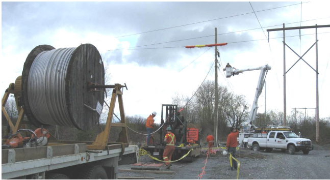
The west end of the pull.
