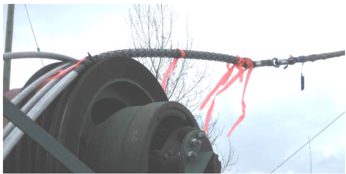
Conductor, grip and line swivel spooling off the tensioner.
