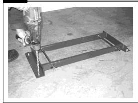
Use only concrete inserts with an ultimate pullout force of 8,000 lb. ensure that they are installed in accordance with the instructions provided by the insert manufacturer. Failure to do so may result in death or serious injury.
